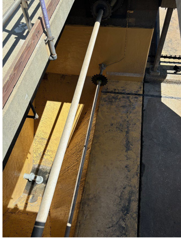
Repaired and Coated Sludge Hopper
