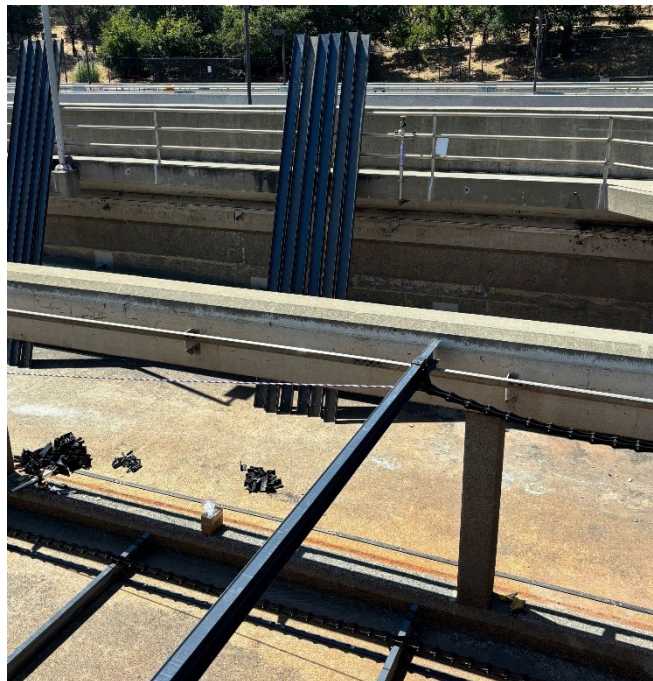
Installing New Flights and Chain in Primary Clarifier No. 1
